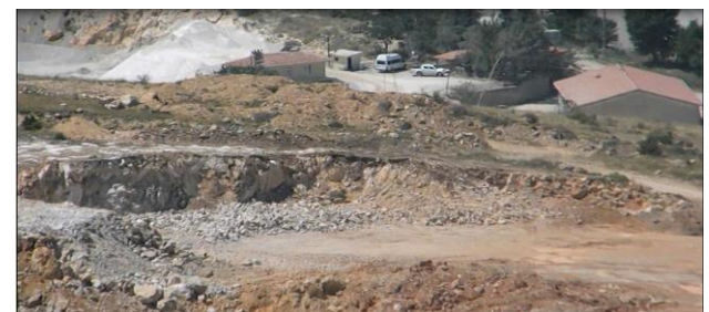
Figure 3. The view of Çorum Municipality's building site
