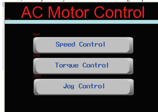
b) HMI control panel
